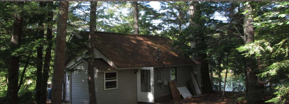
Proposed demolition for elevated house.
