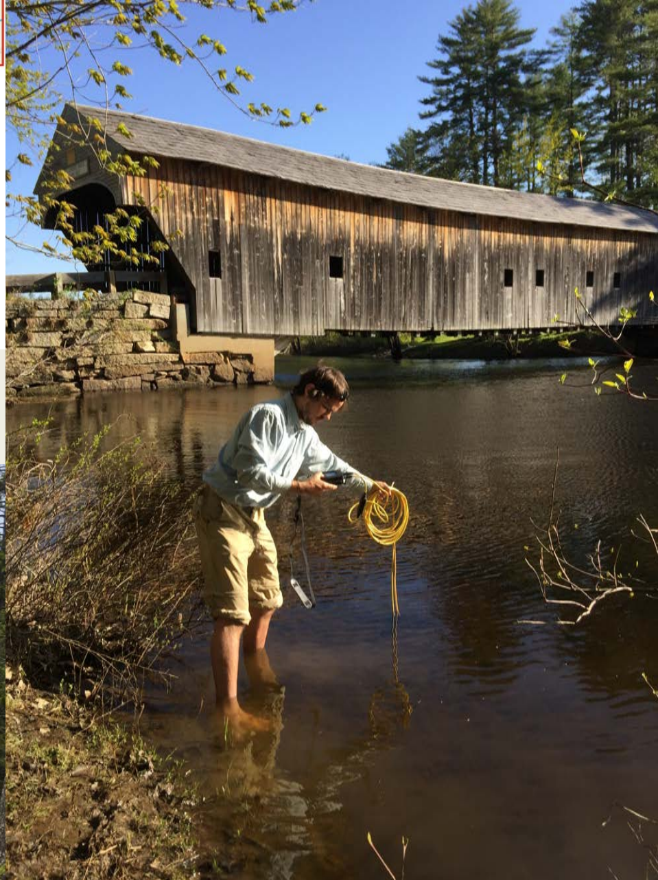
Site OCS4-B: Hemlock Bridge, the Old Course Saco River. Fryeburg, Maine.
